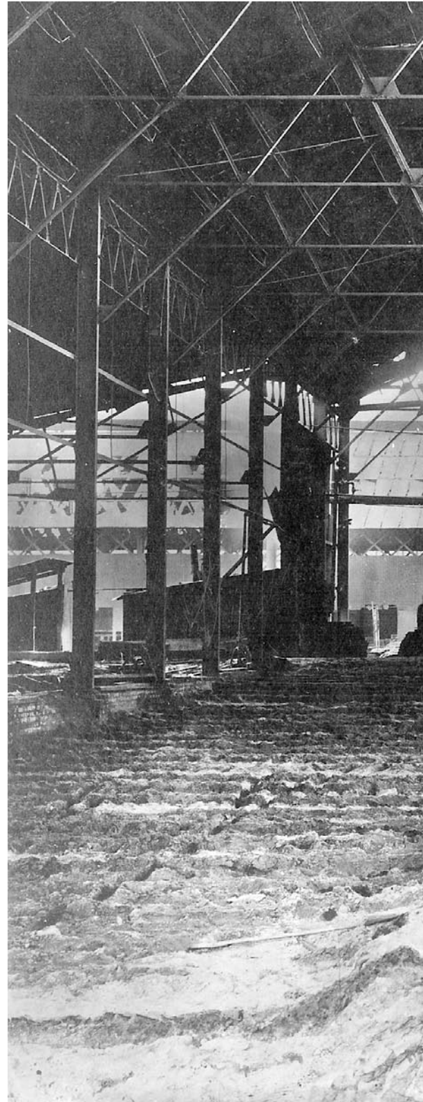
The casthouse for this turn-of-the-century furnace located at Birmingham, Alabama, was similar to the casthouse at the Johnson City furnace. The base of the furnace can be seen at the far end of the casthouse. The floor of the casthouse is sand and workers use special tools to make depressions in the sand, which will form the pigs once the molten iron flows from the furnace.
